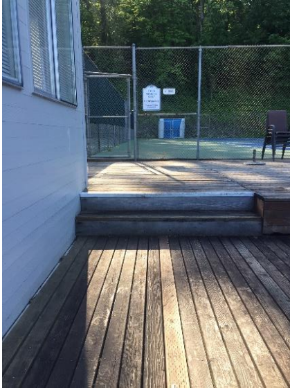
Enter courts via staircase. (East Side)
